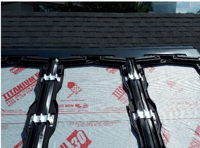
Adjustable frames that can accommodate different PV-panel sizes.
